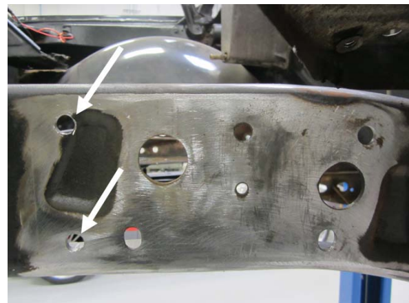
Drivers Side Wheel Well, Drilled Holes
