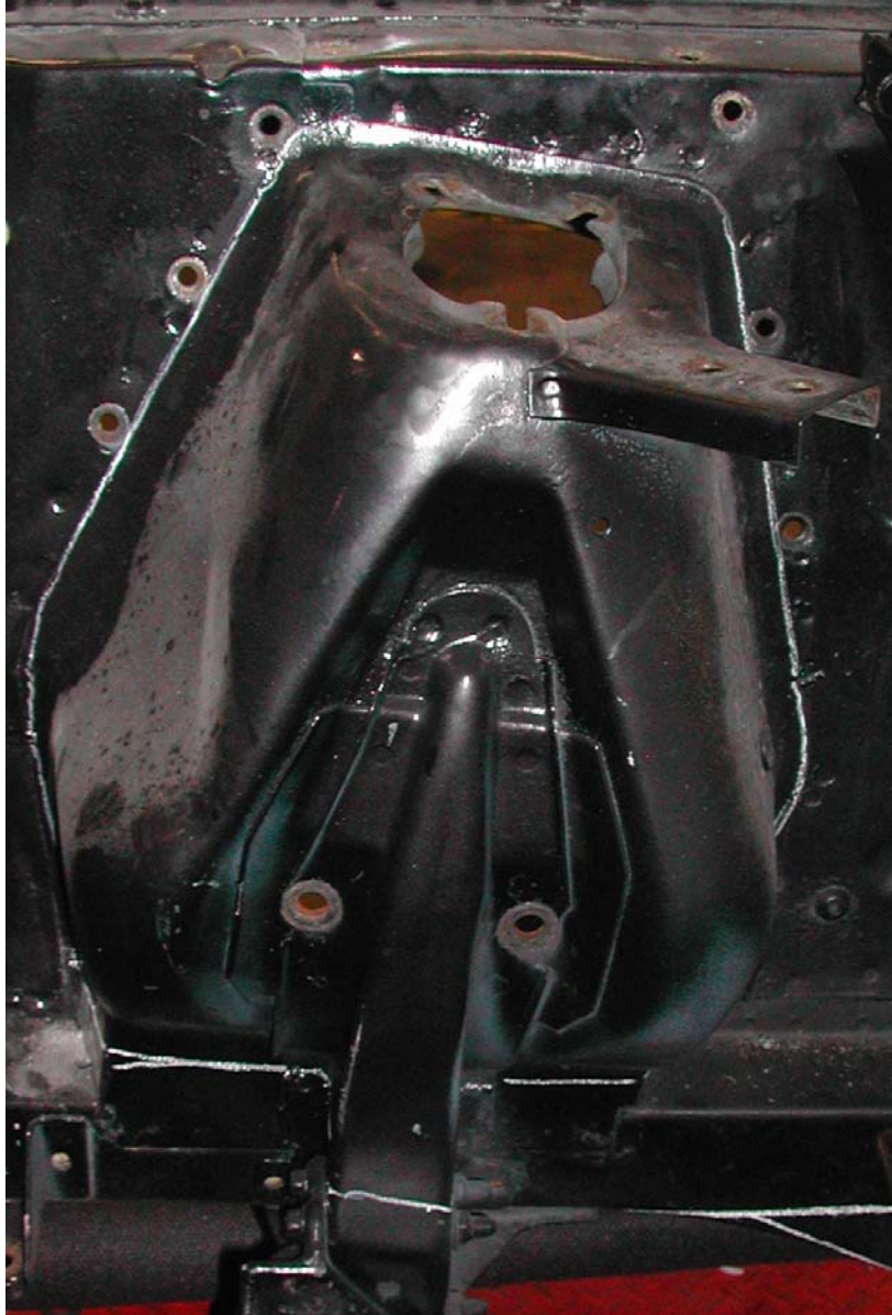
Figure 1. Cut line around Passenger Side Shock Tower
